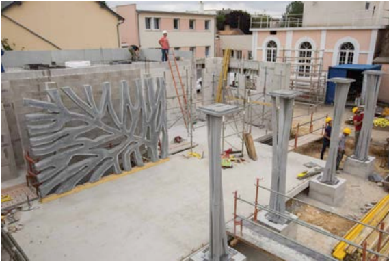
Fig. 49 Moulds for 3D printed outdoor columns.
