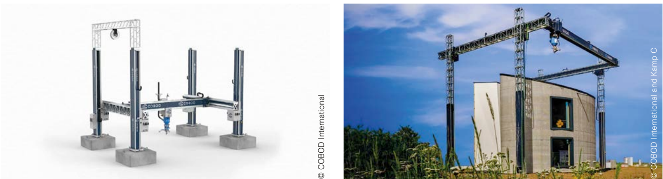
Fig. 46 BOD2 printer (left) and house printed using BOD2 at Kamp C (right).
