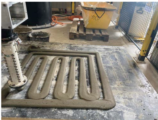
Fig. 18 Printed mortar based on recycled sand from Belgium supplied by the RECYMEX non-hazardous waste recycling centre (experiment conducted at Buildwise in collaboration with ULiège).
