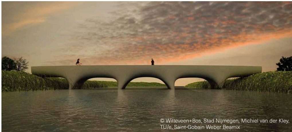
Fig. 59 3D printed footbridge in the Netherlands.
