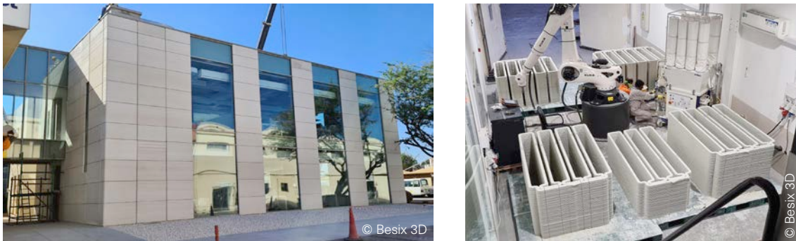
Fig. 55 3D printed mortar façade.
