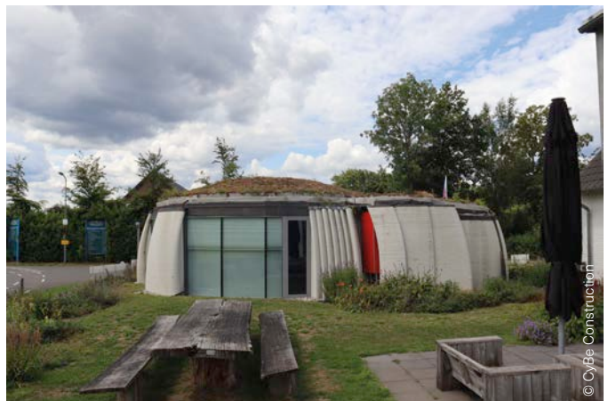
Fig. 43c Printer CyBe RT (Robot Track) and example of a printed structure in the Netherlands made by robotic printer CyBe RC – https://cybe.eu/ .
