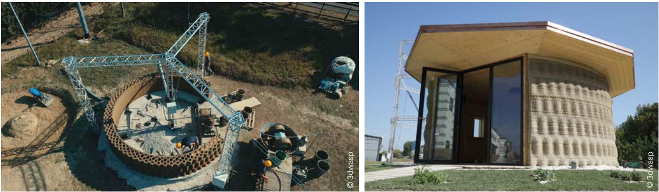
Fig. 16 Gaïa house printed using the Crane WASP printer.
