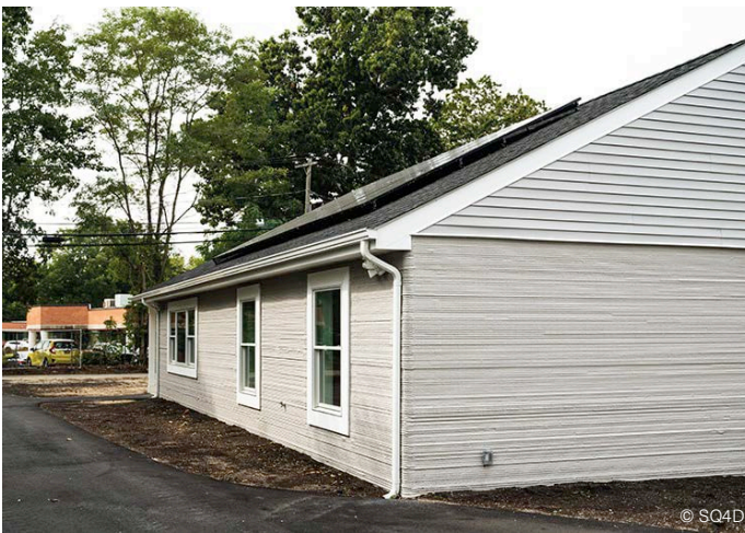
Fig. 13 House printed by SQ4D.
