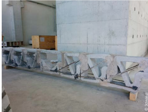
Fig. 30 Beam reinforced through assembly by external reinforcement.
