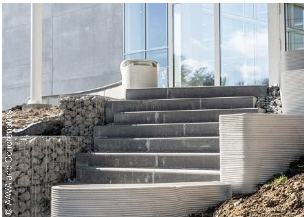
Fig. 54 Printed elements surrounding the outdoor staircase at the new building of Buildwise in Limelette.
