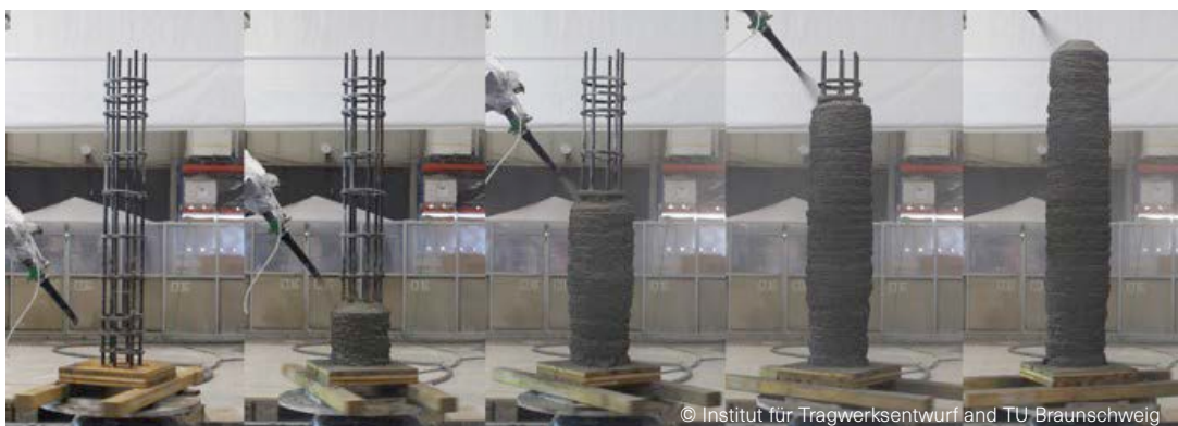
Fig. 29 Stages in building a reinforced column using the SC3DP method.
