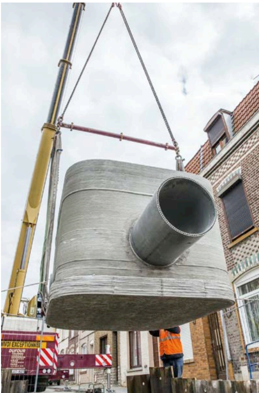
Fig. 50 Stormwater overflow installed in La Madeleine, Lille, France.
