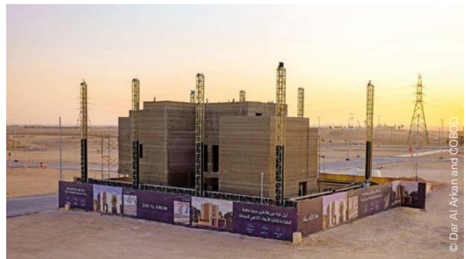
Fig. 34 3D construction projects undertaken using COBOD printers. Office printed under a tent in Denmark (left). Three-storey house 3D printed out in the open air in Saudi Arabia (right).
