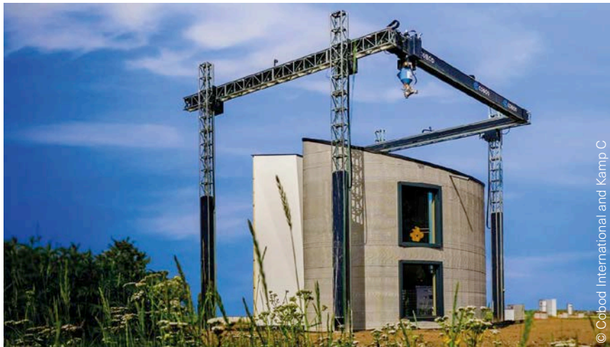
Fig. 10 Two-storey printed house at Kamp C in Westerlo.
