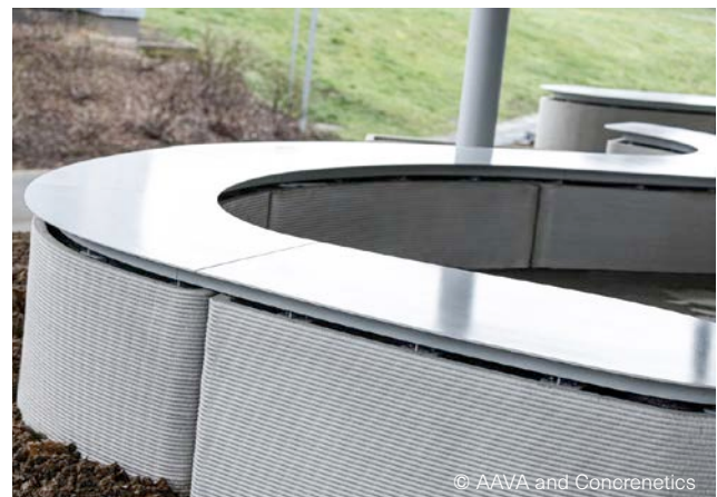
Fig. 54 Printed elements surrounding the outdoor staircase at the new building of Buildwise in Limelette.
