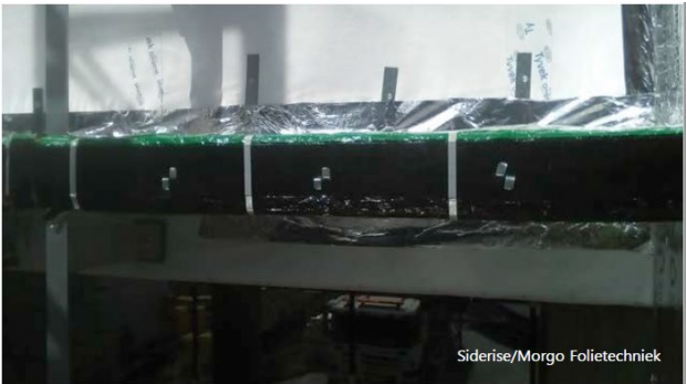
Figure 38 – Application of an intumescent strip in a ventilated facade.
