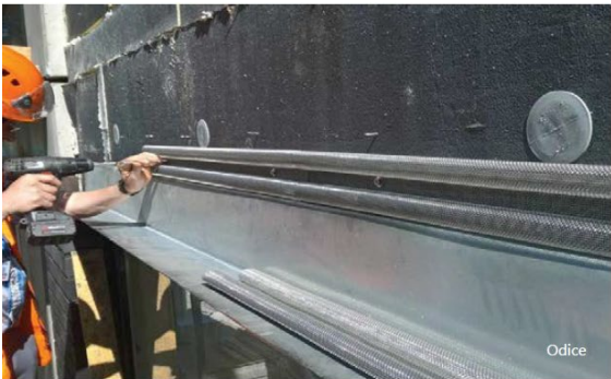
Figure 38 – Application of an intumescent strip in a ventilated facade.
